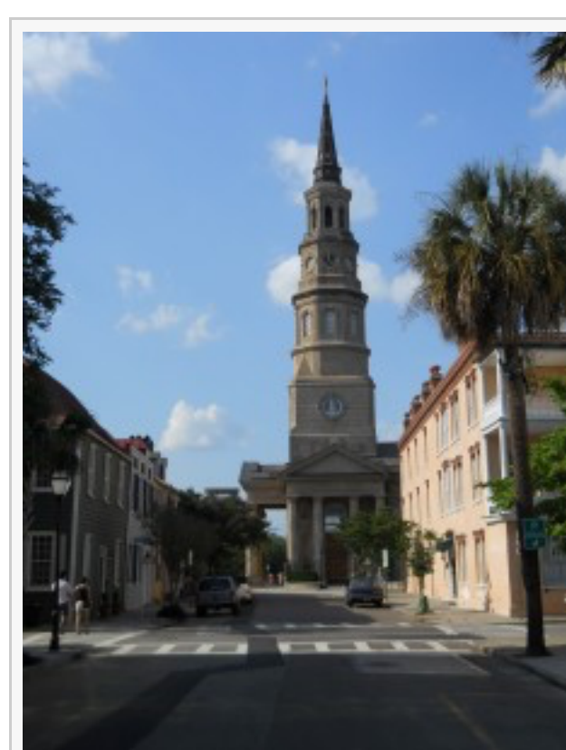
Figure 1. Charleston, SC. The consistent scale, styles and character of Charleston's historic district are today threatened by inappropriate new buildings that introduce alien kinds of architecture. The proposed building for Clemson University's architecture programs was withdrawn in the face of public opposition, but that and other projects continue to be approved by the city's Board of Architectural Review, which has been eager to promote "the architecture of our time." But what is a historic district for? All photos by the author
