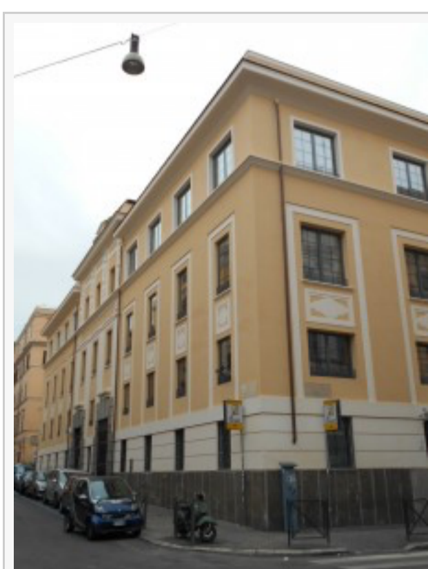
The new home of the University of Notre Dame School of Architecture Rome Studies Program in the Celio neighborhood one block from the Colosseum. The newly renovated early-20th-century building includes studios, classrooms, library and other academic facilities, as well as a host of technological tools to facilitate learning. All photos by the author.
